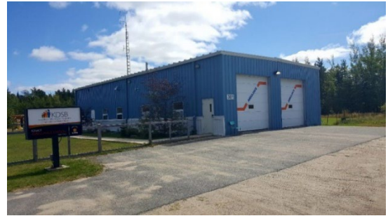
Figure 3-11: Northwest EMS Ignace Ambulance Base (KDSB, 2022)
