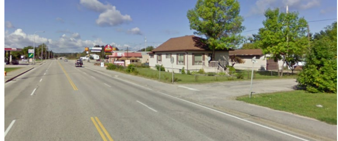
Figure 3-1: Intersection of Highway 17 / James Street Looking West (Source: Google Street View)
